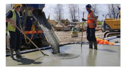
The system requires the contractor to dapple the surface in both horizontal planes to create a smooth finish which is the finished floor level.
